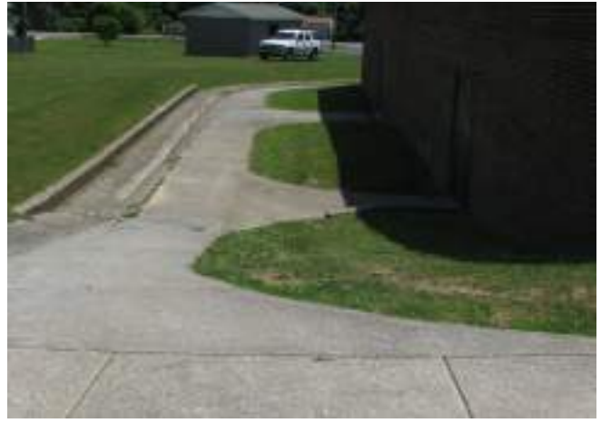
The side basement access is very steep and should be studied for ADA compliance.
